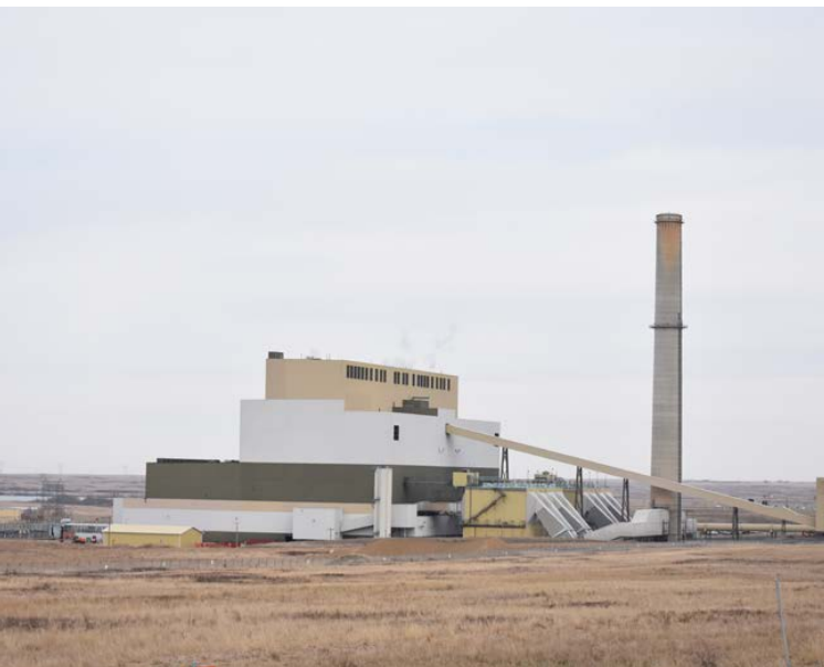
SHEERNESS GENERATING STATION, ALBERTA PHOTO TONYGLEN14/FLICKR
