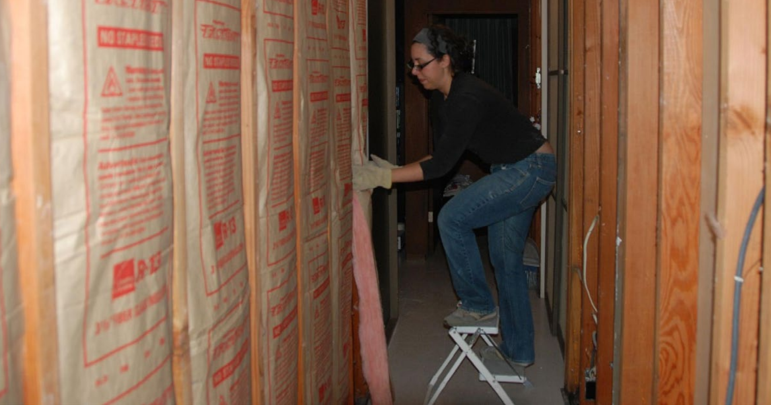
A woman installs wall insulation. Photo by Nick Nguyen (CC BY-SA 2.0).
